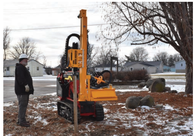
Installing 3" Round Wood Fence Post.
