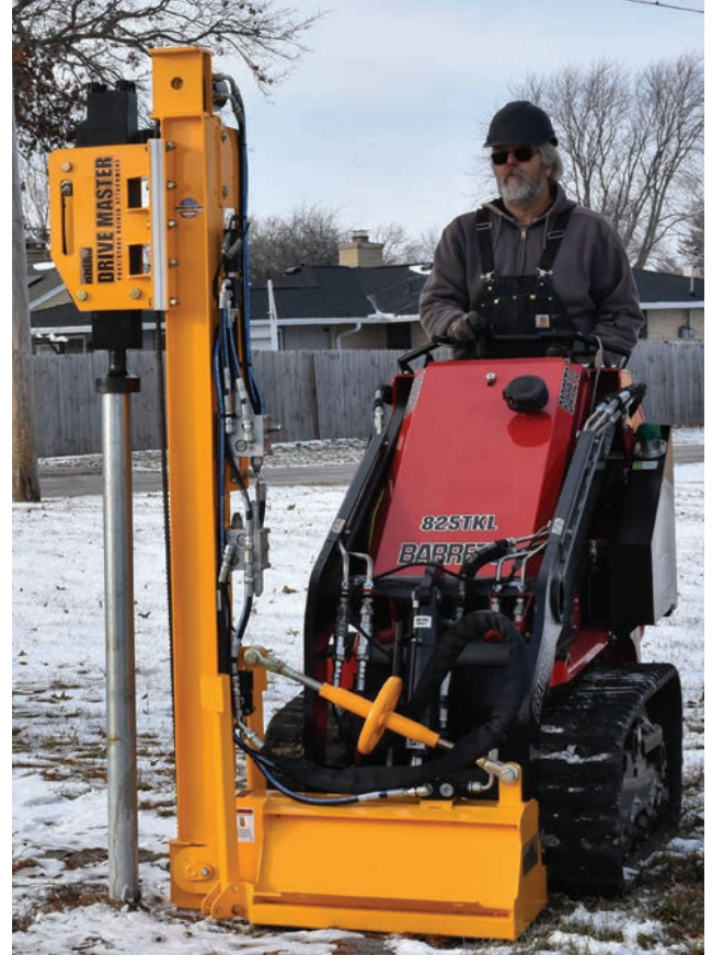
Installing 2 3/8" Terminal Fence Post.
