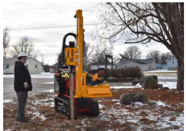
Installing 3" Round Wood Fence Post.
