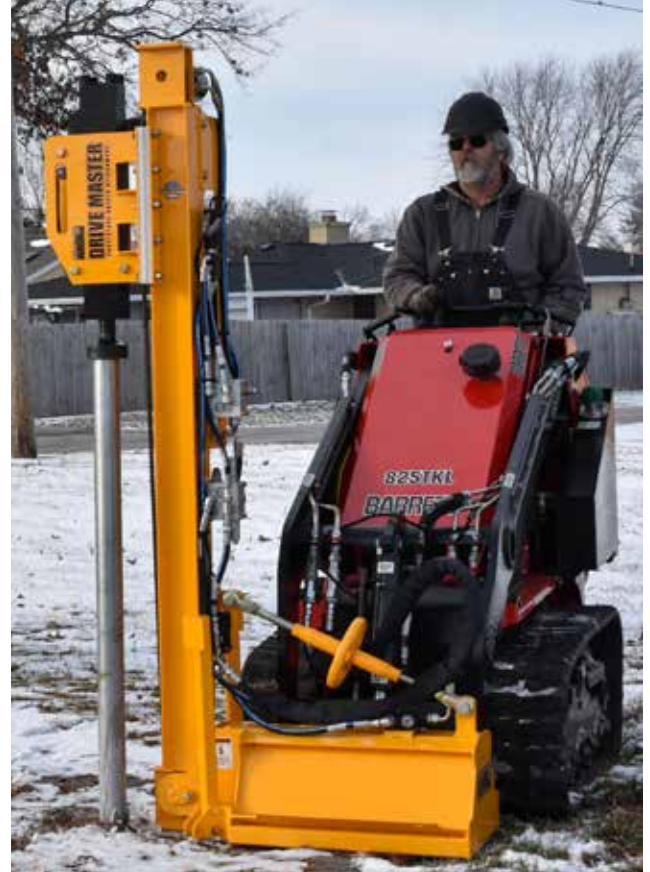
Installing 2 3/8" Terminal Fence Post.
